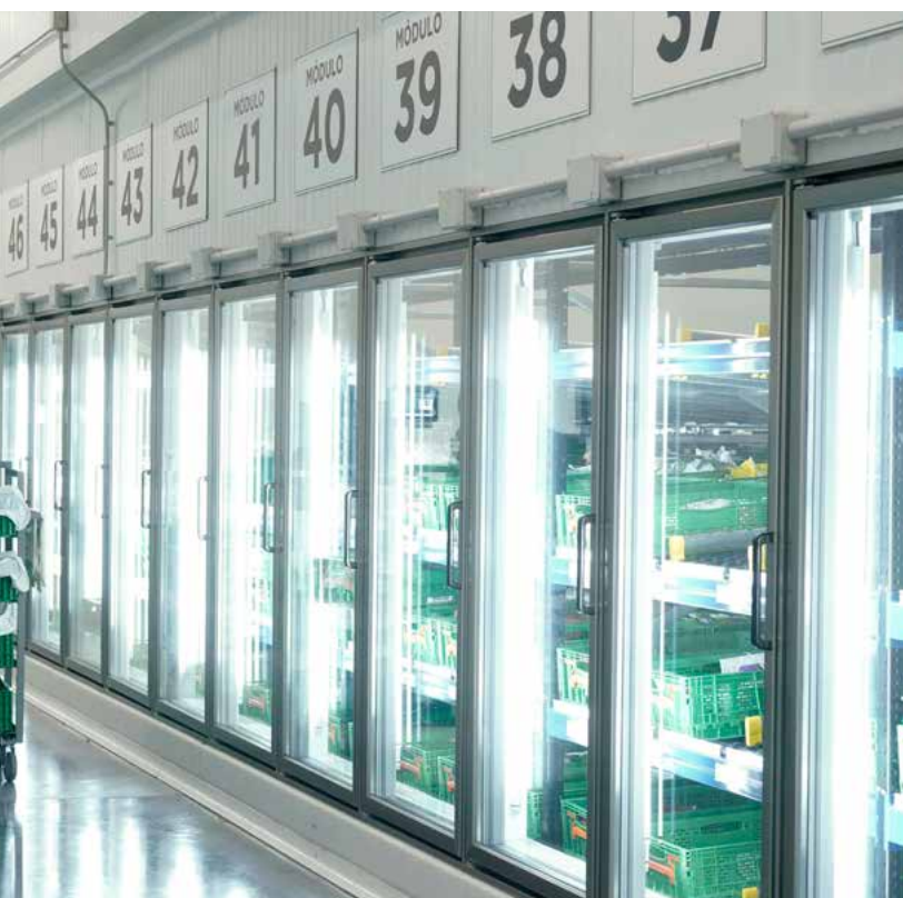
Facilities inside the Hive in Madrid, Madrid.
