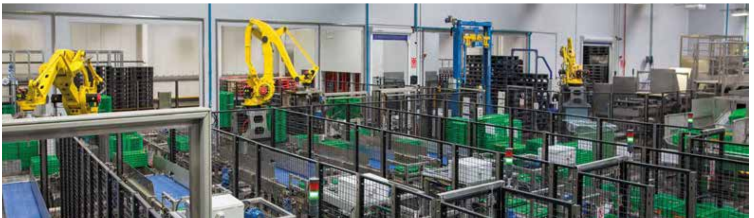
Facilities of the logistics centre in Abrera, Barcelona.
